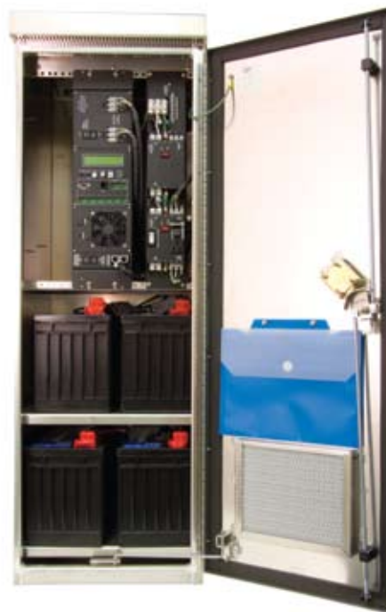
Shown with Alpha UPS module, transfer switches, and AlphaCell batteries.
