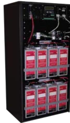
Shown with Alpha FXM 2000, Alpha transfer switches, and AlphaCell™ batteries.
